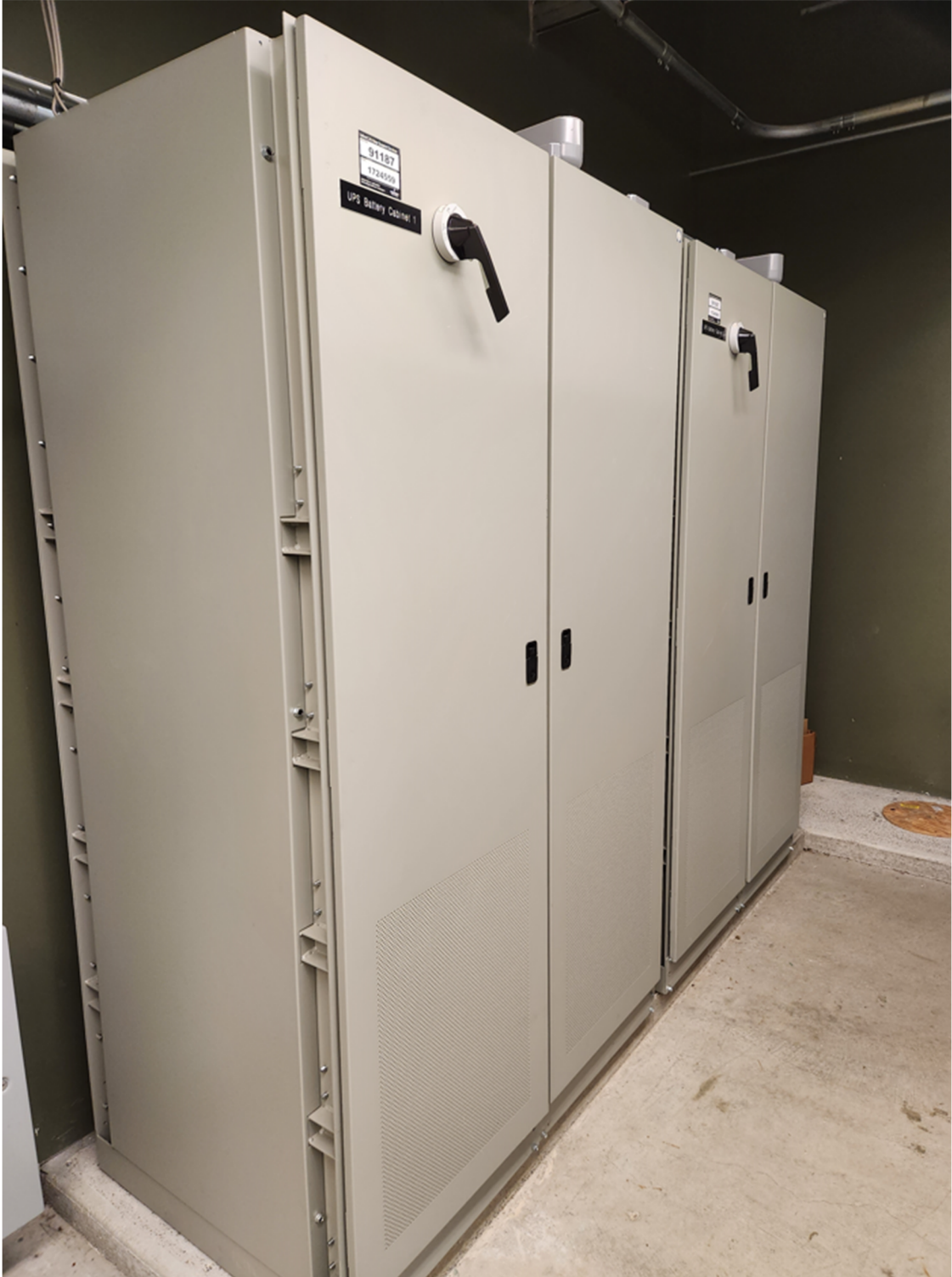
Figure 6: Battery Cabinets
