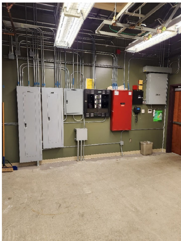
Figure 25: Photo 12 Northwest Wall
