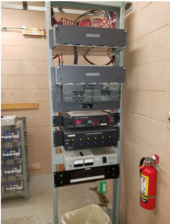
Figure 3: E30 th DC Power Rack and Battery System
