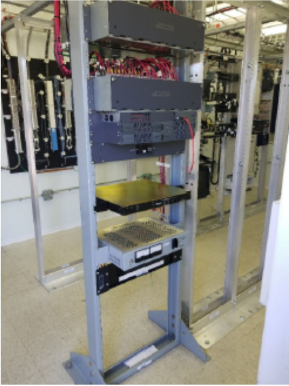
Figure 14: Newberry Hill DC Power Rack and Battery System
