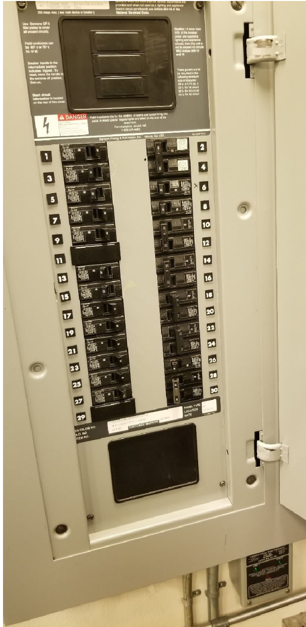
Figure 13: Mandus Olson 120/240VAC Breaker Panel and Circuit Directory (Note: 20A 2P Rectifier Circuit Breakers)
