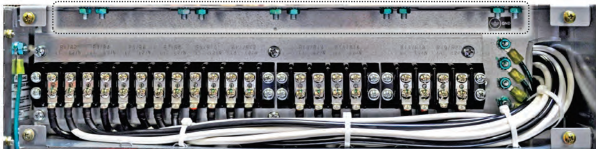
Figure 6 - AC Ground Connections
