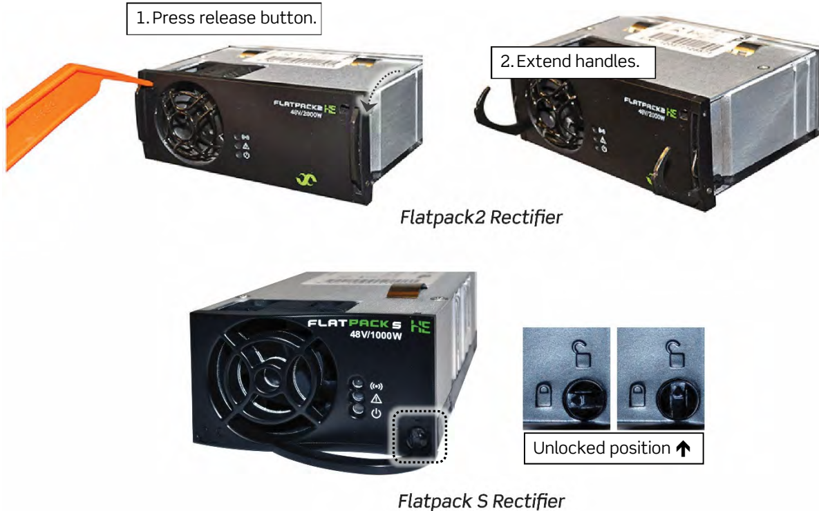
Figure 43 - Unlocking Modules
