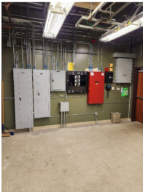
Figure 29: Photo 12 Northwest Wall
