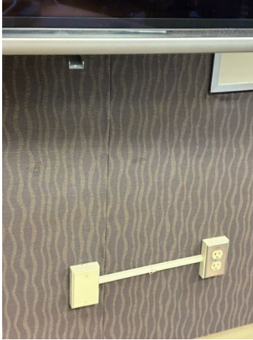
Photo 4 North Wall Close up. The existing outlet under the larger TV monitor on the north wall has an extension junction box. The bid should include hiding this if possible. The existing wall covering would be removed and the underlying drywall will be exposed prior to work commencing.
