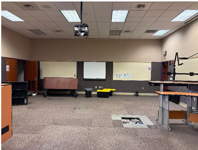
Photo 7: Classroom West Wall. The smart board in the middle is covering an outlet that may be able to be reused for the new monitor. A second outlet on the wall is intended for this wall as well.
