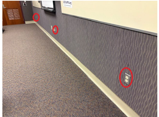
Photo 8: Classroom West Wall. The existing outlets are circled in red and are at standard 16" height.
