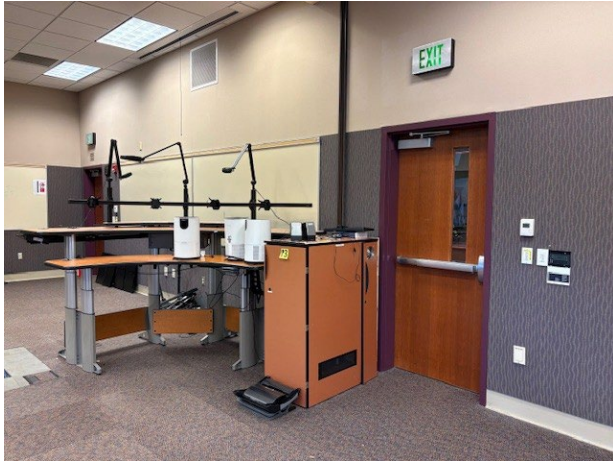
Photo 3. North Wall Part A. The accordion door track that it anchors to when extended can be seen in the center of the photograph. This track is mounted on top of the existing sound dampening panels and likely we will cut away the existing panels rather than taking down the track but this is yet to be finalized.
