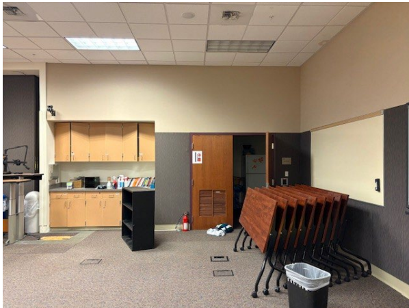
Photo 2: West Wall Part A. All white boards, AV equipment and purple-gray sound dampening fabric and panels will be removed.
