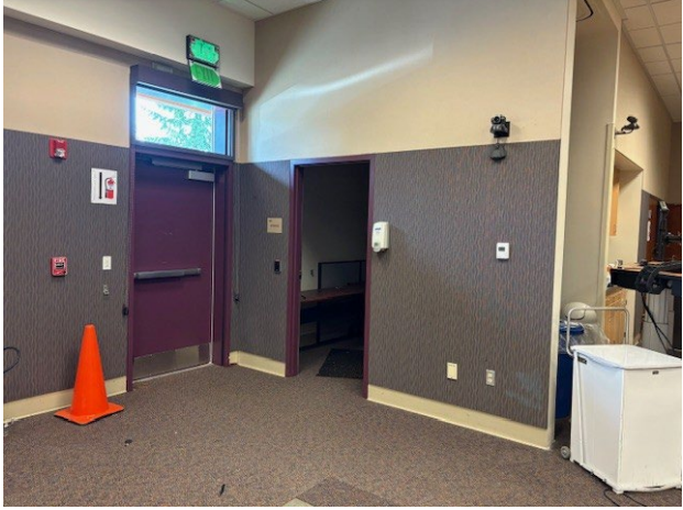
Photo 7 West Wall Part B
