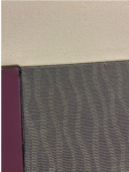
Photo 8: Current Transition. This is the current transition between the upper fabric panels and the lower panels we want to replace with felt and new black tracking.
